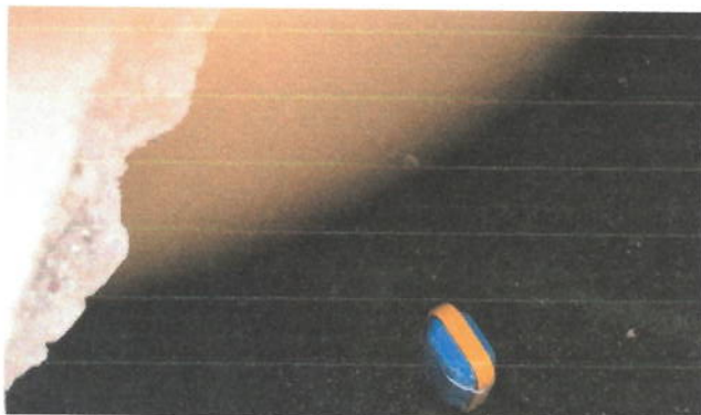
Photo. Sensor placed in overhead water tank
