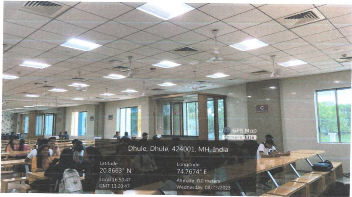
Photo. LED lighting in canteen
